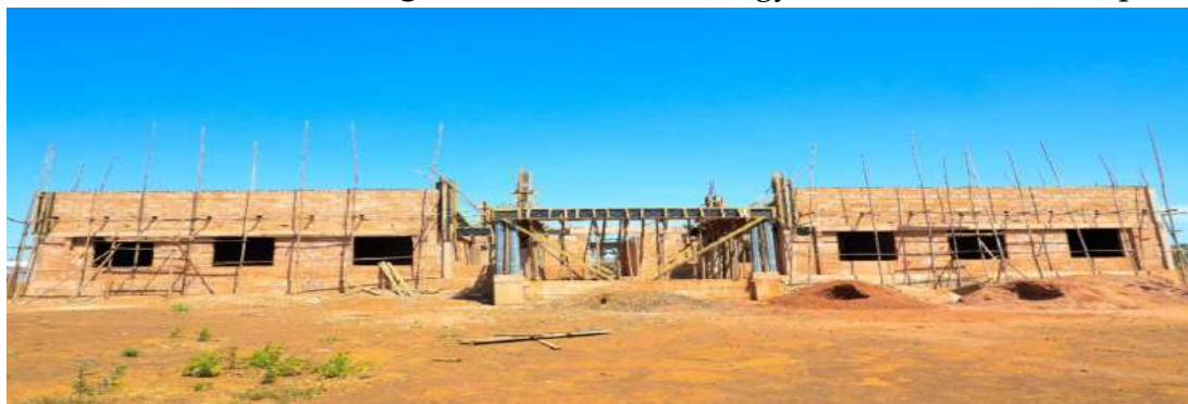
Construction of Kasulu Technical College
