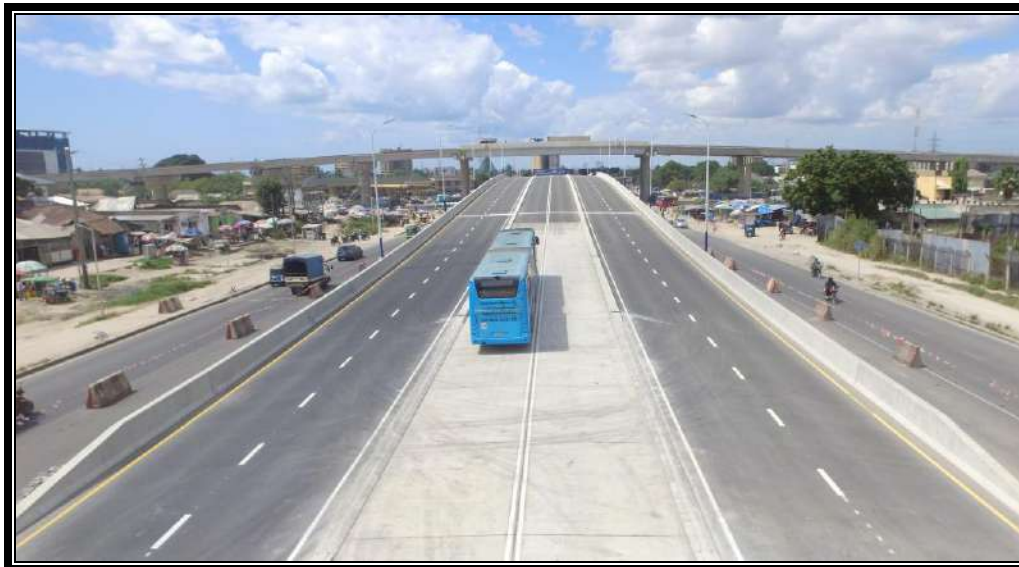
Ubungo Interchange in Dar es Salaam.
